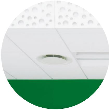
● Replacing the air inside the building 2.5 times as often as in an ordinary office building ensures an optimal indoor climate with efficient ventilation, where pollen and diesel particles from the nearby railway are vented out. This is good for everyone and especially important for employees with allergies or asthma.
